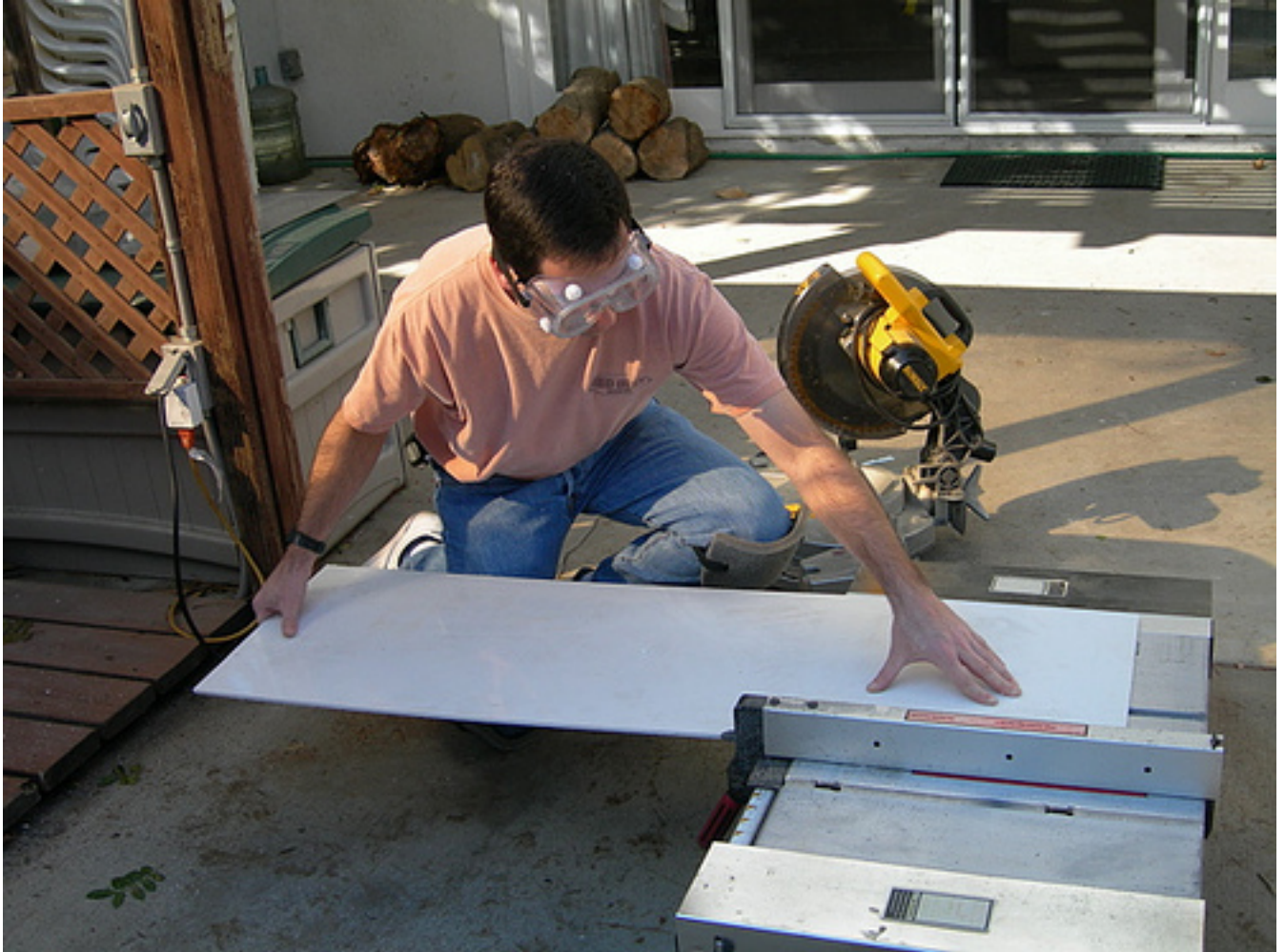
Mike chopped the strips, which were about 4' long, down to size on the miter saw.
