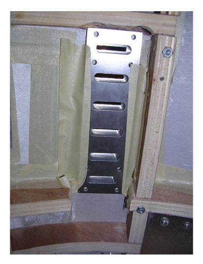
I also had to widen some cuts to the frame's base plate, to make room for the rear coin returns. Back on May 4 of this year I had cut the frame for the same purpose, but I didn't realize that I had reversed the left and right returns. Now that I've fixed that, I had to gouge out some more material.
